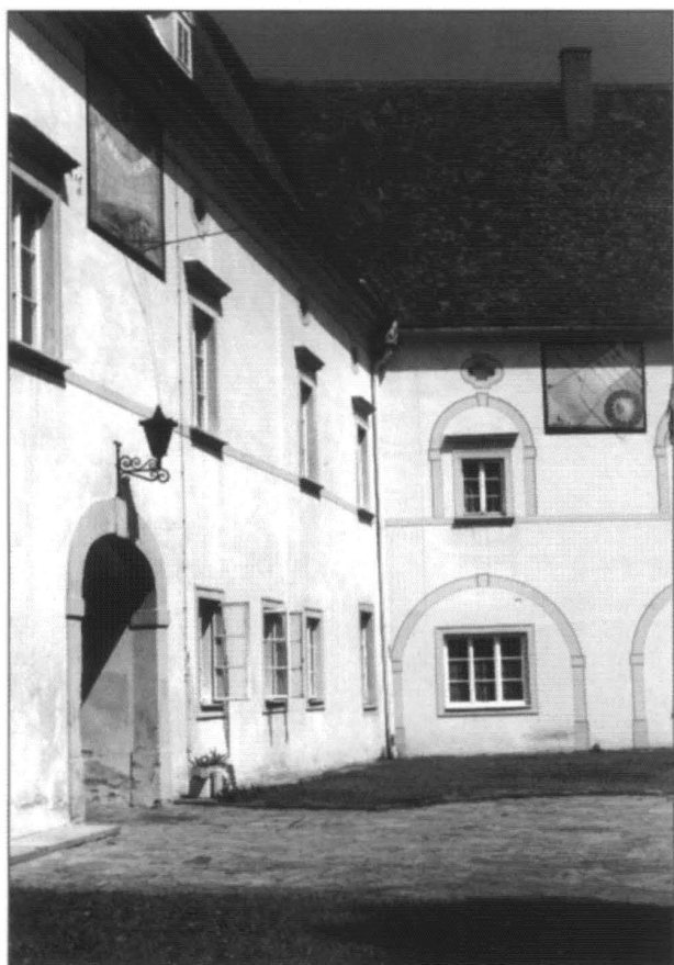
Two of the painted wall-dials at Stift (monastery) Altenburg
