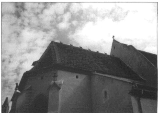
Hares along the roof-ridge, St Michaels Church, Weissenkirchen
